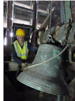
The bells are sent to Whitechapel Bell Foundry to remove the canons (old-style fixing points on top of bells), send them off to be sandblasted clean of corrosion, and then skilfully re-tune each bell. The bells continue their journey to Nicholson's in Bridport, Dorset to be assembled in the newly fabricated frame.
