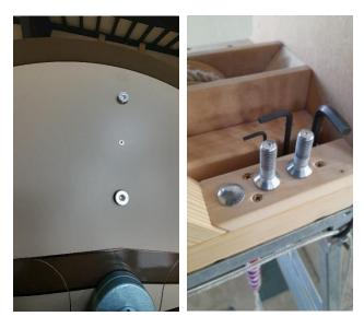
Now that the stay is functioning, the wheel can be rotated until the fastenings for the bell weights are at the top (just like it will be when the bell is rung up).
